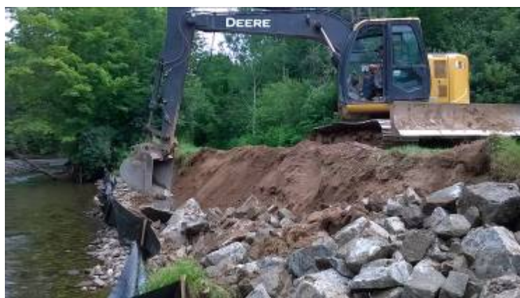
During work in the summer of 2015, rock was placed by an excavator.
